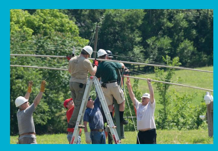
Taking the antenna and a small mast off of the rotor
