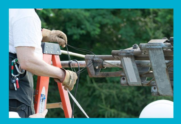
N4PD uncoils the coax and his helper lays it on the ground in an S shape. This allows the tower to be raised with minimal risk of the coax getting kinked.
